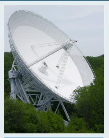
The 100-m diameter Effelsberg antenna (Germany), used during all the VLBI experiments to observe weak extragalactic radio sources for the alignment with the future Gaia frame. The large diameter is necessary to achieve the high sensitivity to detect such weak sources (Picture credit: Dr. Schorsch).
