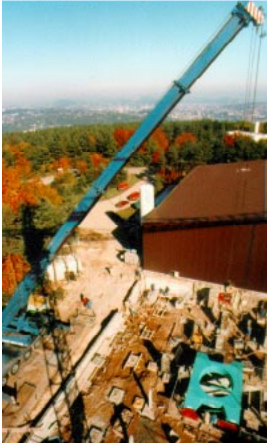
PICTURE 1 : Seismic block installation.
