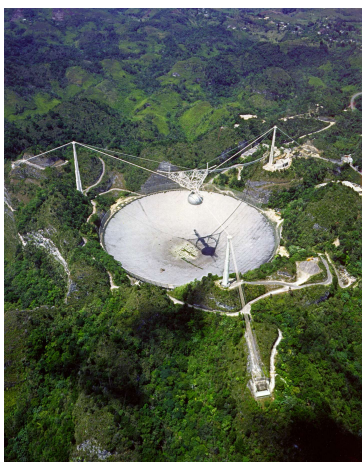
Fig. 8a (left): 305 m diameter Arecibo radar facility (permanently closed since November 2020 due to structural collapse). Fig. 8b (right): Artist's impression of the WISE spacecraft in orbit around Earth. Credit: NASA
