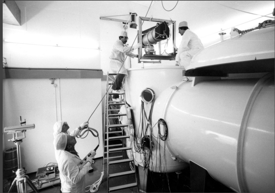
Baumgartner, Heinrich Bräuninger, Robert Giralt and myself lowering the LE-instrument in the Panter facility
