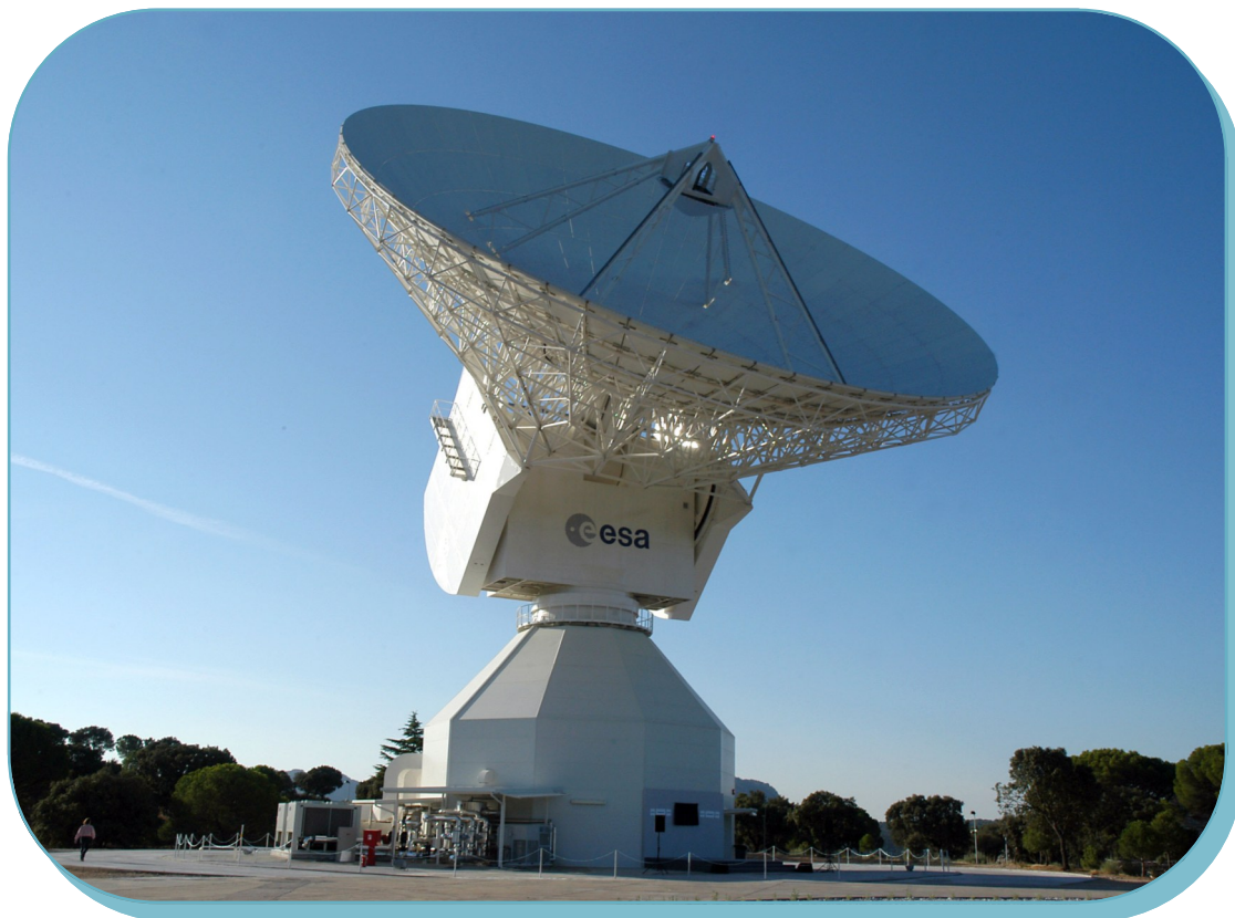
The 35-meter antenna in Malargüe, Argentina, has been completed and officially dedicated last December. This is the new ESA antenna built for communication with satellites in deep space. It will be operational in 2013 and will contribute to the Gaia tracking (even if indirectly by relieving Gaia from the ground station booking pressure). Picture credit ESA.
